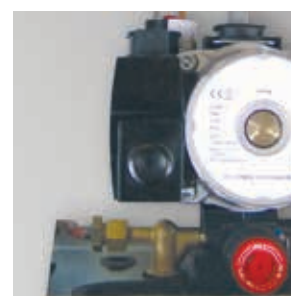
Pump body with built-in air vent
